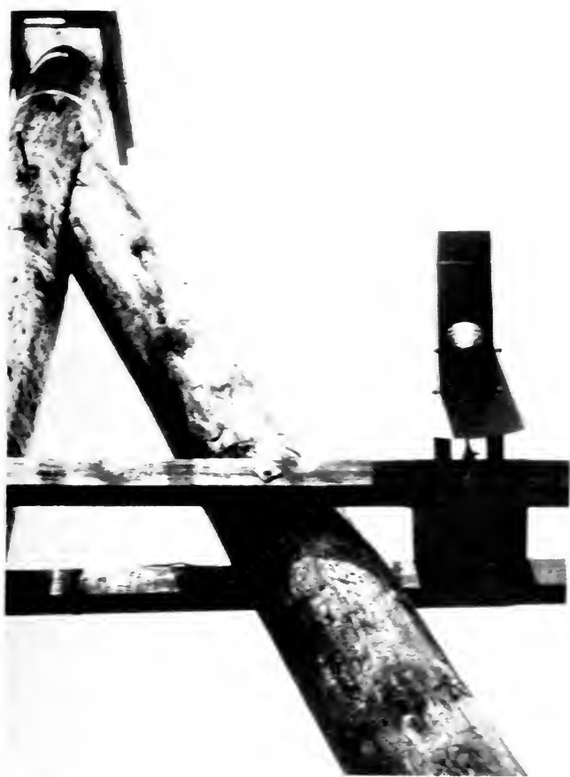
Fig. 4—Another view of photoelectric detector of high and wide clearance.
